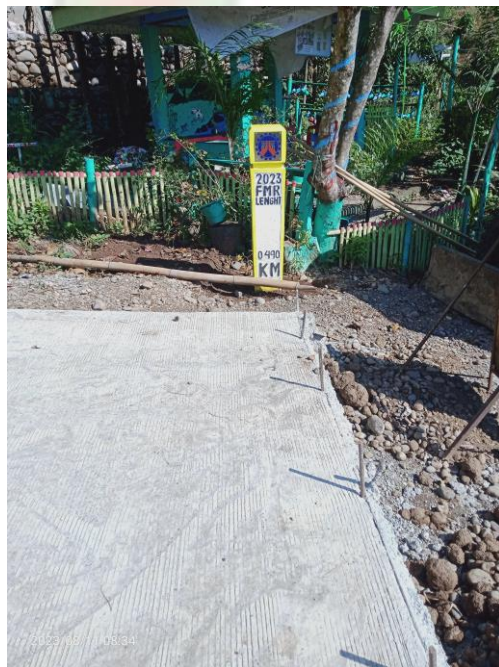
Construction of Farm to Market Road at Purok 1 Calaoacan
